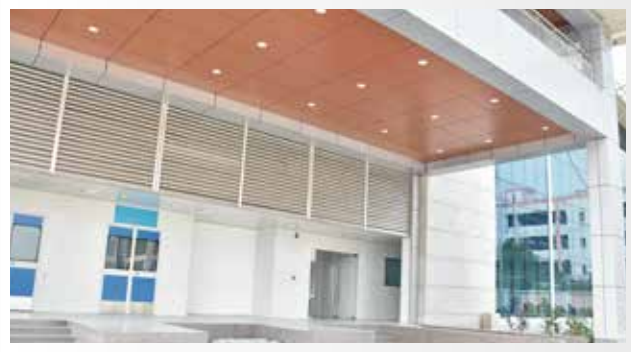
Entrance of Production Building
