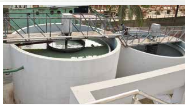
Effluent Treatment Plant
