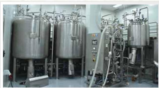
Liquid Manufacturing Vessel
